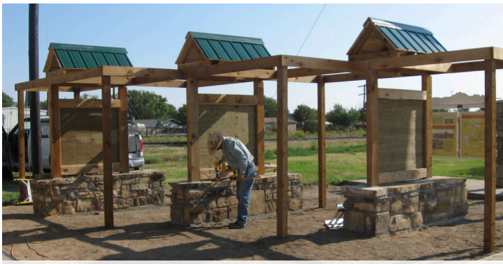
Example amenity site with three interpretive sign panels, shown under construction.
